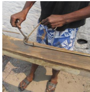
How is this for hand-molding rebar!
